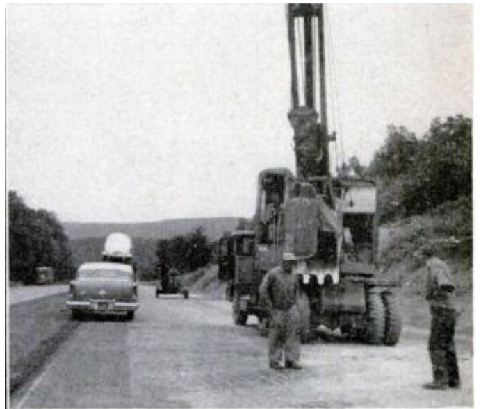
ROAD REPAIRS flagged us down, too. All told, we had eight miles of one-lane traffic.
