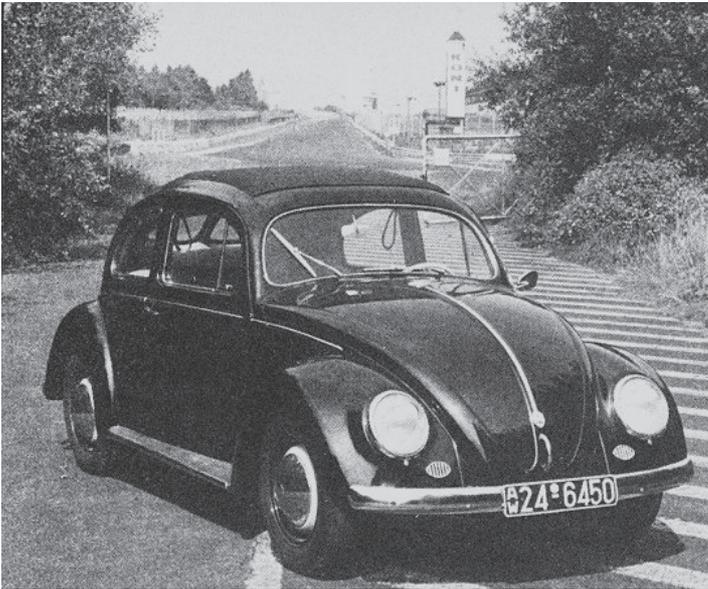
Volkswagen actually commissioned an air-cooled, flat-four Beetle-based diesel from its regular future projects supplier, Porsche, way back in 1951. This was given Project Number 508, and carried on to making one test vehicle and two test engines. The project even provided vital strength data for Porsche's own 1.3/1.5-litre crankcase, but it would be 1981 before the public learned about this decidedly different VW engine. Among those 21 million-plus Beetles, only one was destined to be a diesel.
