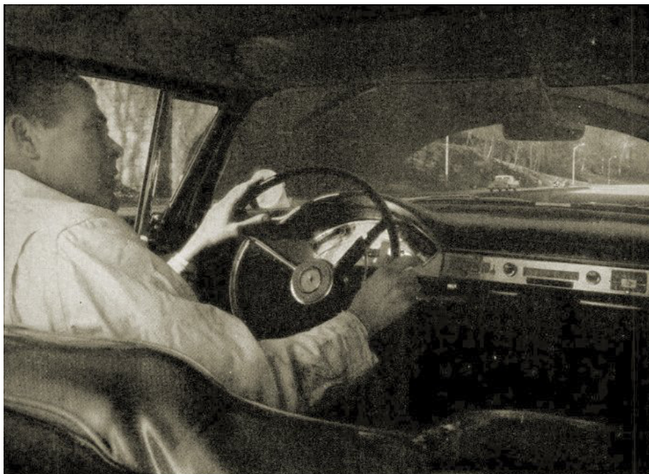
"Most car noises can be checked best with all car windows closed," says Stronsick. "But I also drive through an underpass—the longer the better—with the driver's window open. That way I hear noises reflected from under the car."
