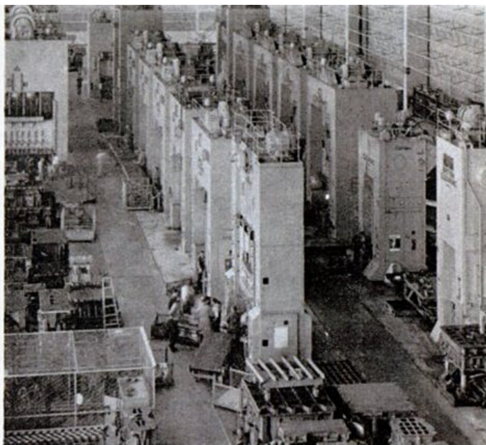
The huge press shop at the Clayton plant. Sheet steel is stored at the far end of the building, then is stamped into shape in the banks of presses.
